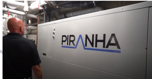
Wastewater Energy Exchange
