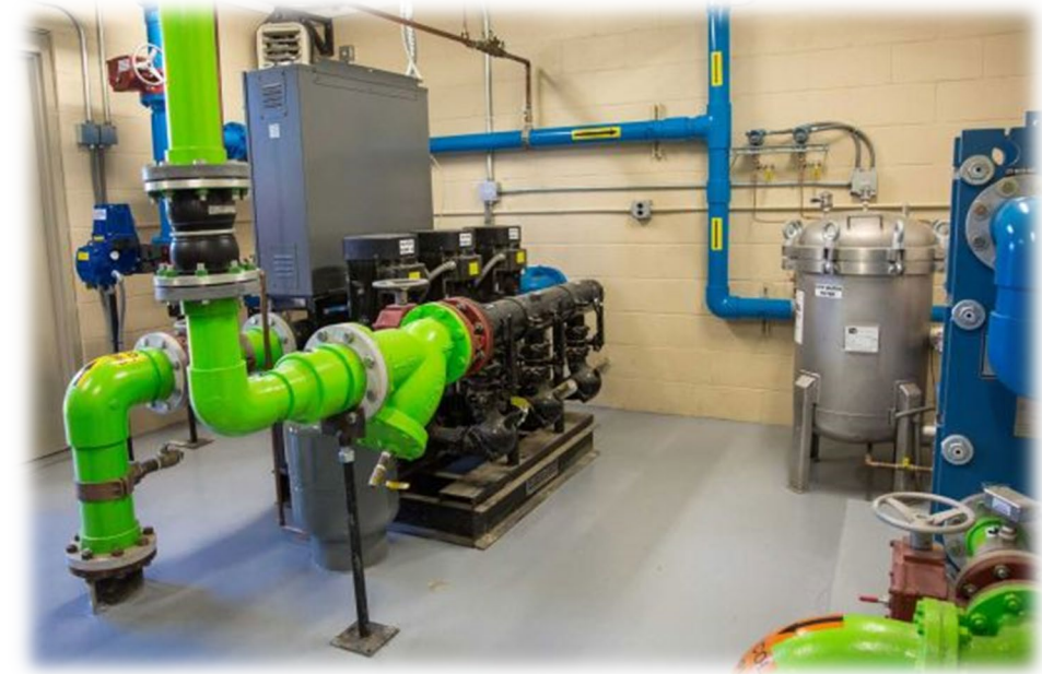
Geothermal Heat Pump (Left) and Exchanger Room (Above)
