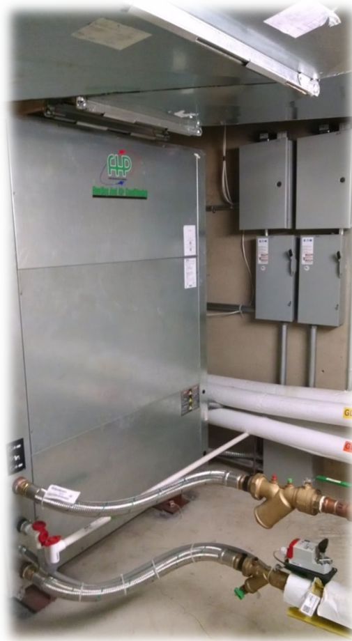
Geothermal Heat Pump (Left) and Exchanger Room (Above)
